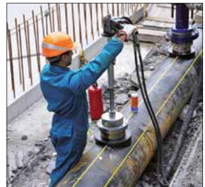
AH15 in action on typical pipe drilling/hot tapping equipment
