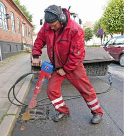
The advantage of hydraulic breakers is that they can be connected to the hydraulic takeout on the various machines of the asphalt companies. This way it is easy to connect the breaker and get the job done and then move on to the next machine job. Therefore most of the asphalt companies have mounted a breaker ready for use at the side of the machine.
