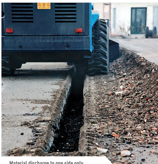
Material discharge to one side only
